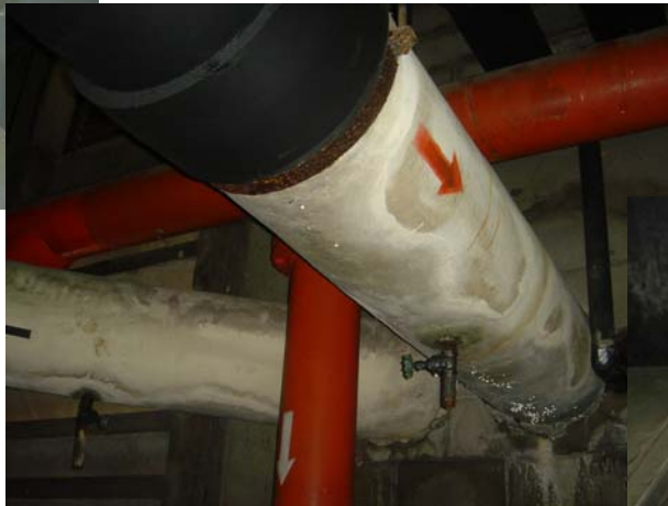
Leakage in the cooling system
