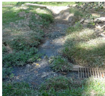
(b) Blockage of drainage system
