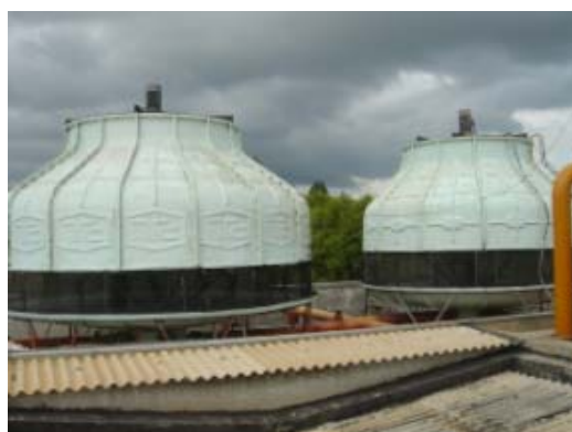
(b) Cooling Towers in Chiller room
