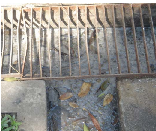
(c) Leachate spills down to the drainage
