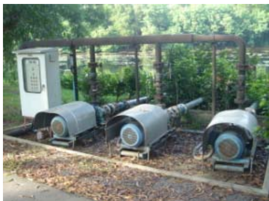
Figure 4.23 Pumps for Gardening Water
