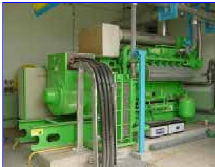
Gas Engine to produce electricity in Biogas Utilization Process
