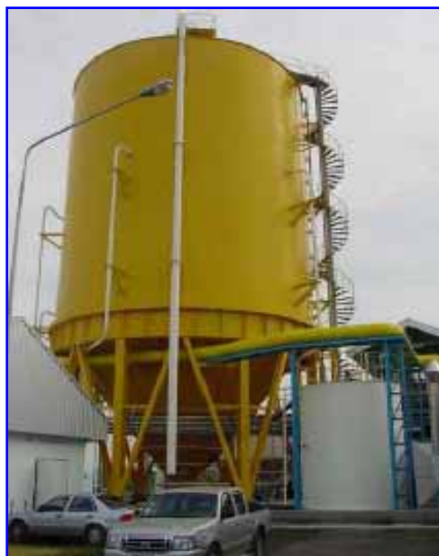
Bioreactor (HLAD Tank) with cap. 2400 m 3
