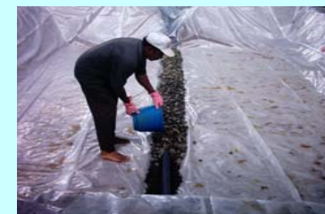
Fabrication and Evaluation of Refuse Polythene-based Landfill Liner
