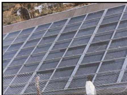
Solar heat panels installed on the roof of a tea factory results in significant reductions in fuel consumption (Source: Palaniappan, 1993)
