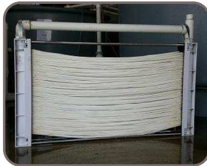
Figure 5 (b) Micro-filtration membrane used in the MBR of the RAS
