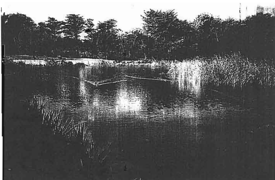
900A macrophyte lagoon, one of a series of three lagoons which serve as the tertiary treatment stage of the wastewater reuse project on the island of Porquerolles, France.
